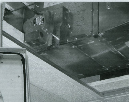
▲ One of three smoke dampers for closing ductwork during a fire.
