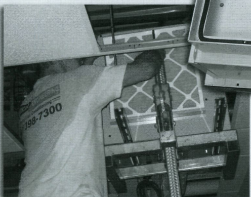
▲ Jacking the dehumidifier up into the hallway ceiling.
