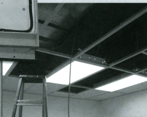
▲ Sealed lighting fixtures and heavy ceiling tiles in grommeted gridwork.
