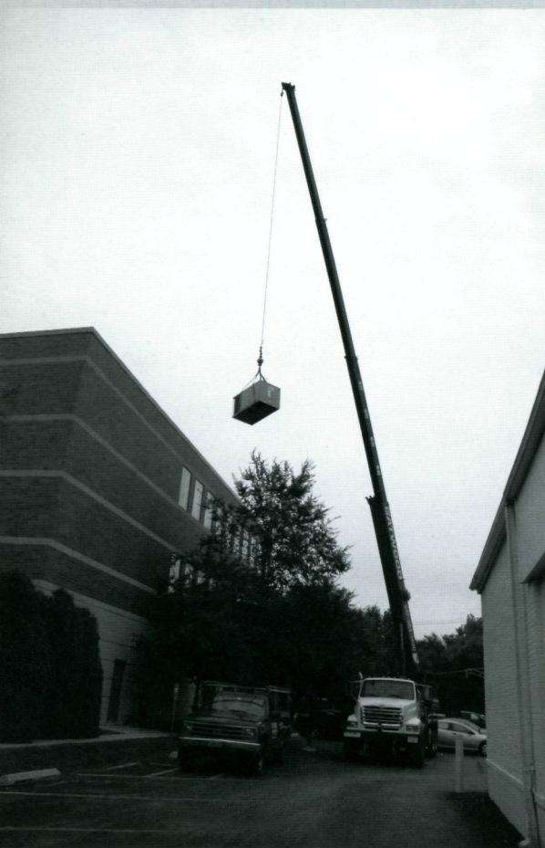
Craning the 2.5-ton air conditioner onto the HVAC penetration through the ASA headquarters building's roof.
