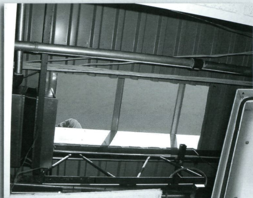
▲ Looking up through the hallway ceiling and out through the roof penetration, awaiting the 2.5-ton air conditioner.
