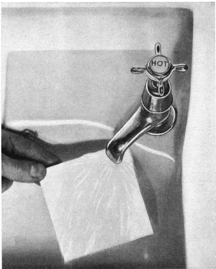
FIG. 6. The tile is warmed under the hot-water tap and dried.
